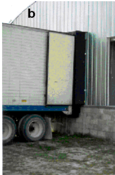
Figure 3. (b) The raised dock permits loading of cooled crops directly from the cold room.
